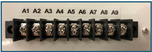
9. For fan interlock to function, place a jumper between A3 and A2. Next, connect terminal A1 on the dehumidifier to the remote fan terminal on the HVAC controller (normally terminal "G").
